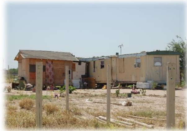
The colonia home shown above is situated on a cinder block structure. Photo credit: Federal Reserve Bank of Dallas, Las Colonias in the 21 st Century report, 2015.
